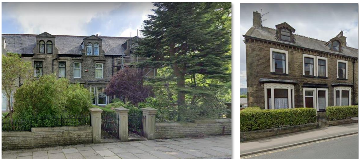
Figure 22: Found on larger period properties in Burnley - Dormers at Rosehill Road and Padiham Road (Courtesy of Google Street View)
