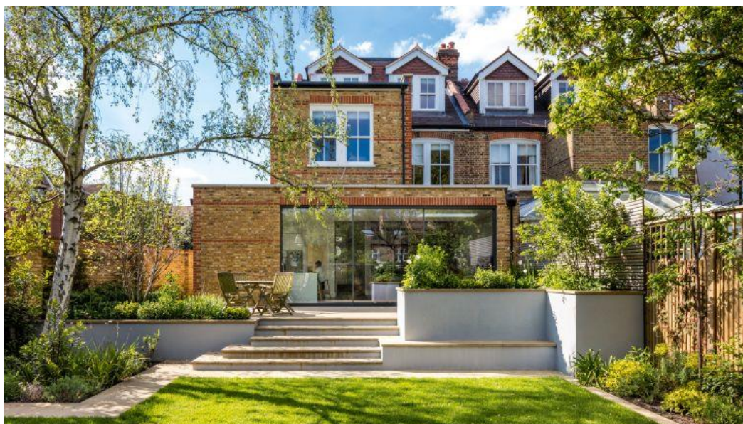
Figure 5: Contemporary/contrasting extension on a traditional style house built using matching brick with quoins, heads and banding detail to match the existing dwelling (Image credit: Grant Architecture and Interiors)
